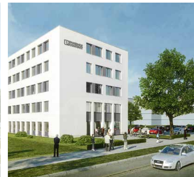
Prototyp: Firmensitz der Phoenix Contact Cyber Security AG, Richard-Willstätter-Straße Prototyp: Head office of Phoenix Contact Cyber Security at Richard-Willstätter-Straße
