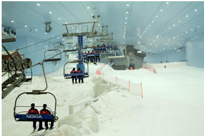
© Polar Refrigeration GmbH –www. polar-refrigeration.de
