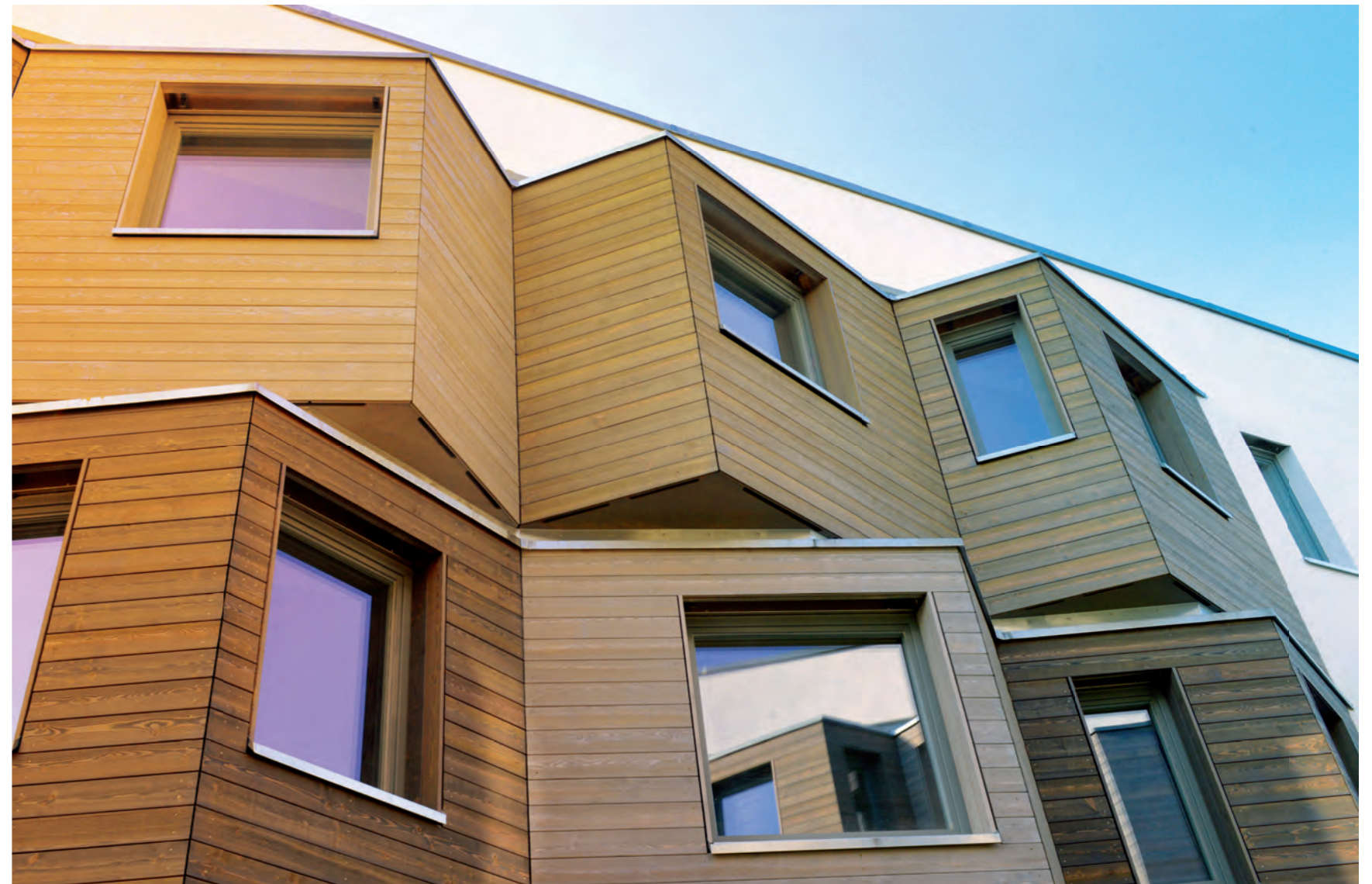
„Denker-Erker“ an der Fassade des Studentendorfs Adlershof Bay windows for concentrated study at the Student Village Adlershof
